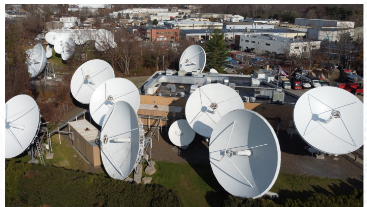
Encompass Glenbrook Teleport; Stamford, CT
